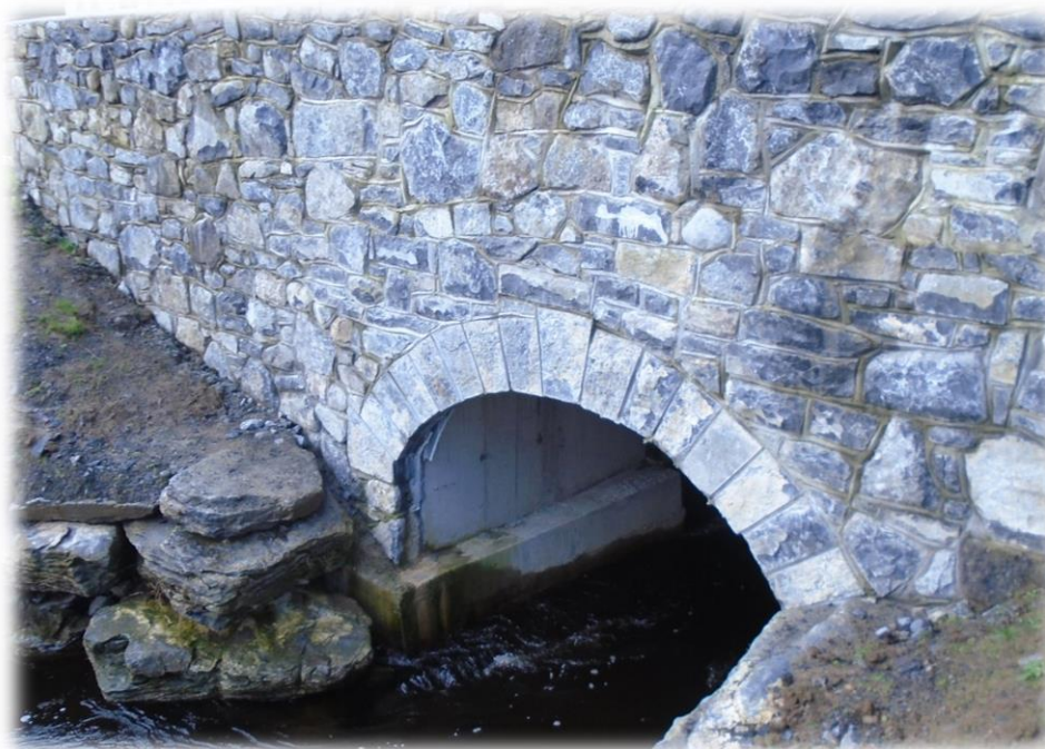
Cloondahamper Bridge, Tuam completed in 2020
