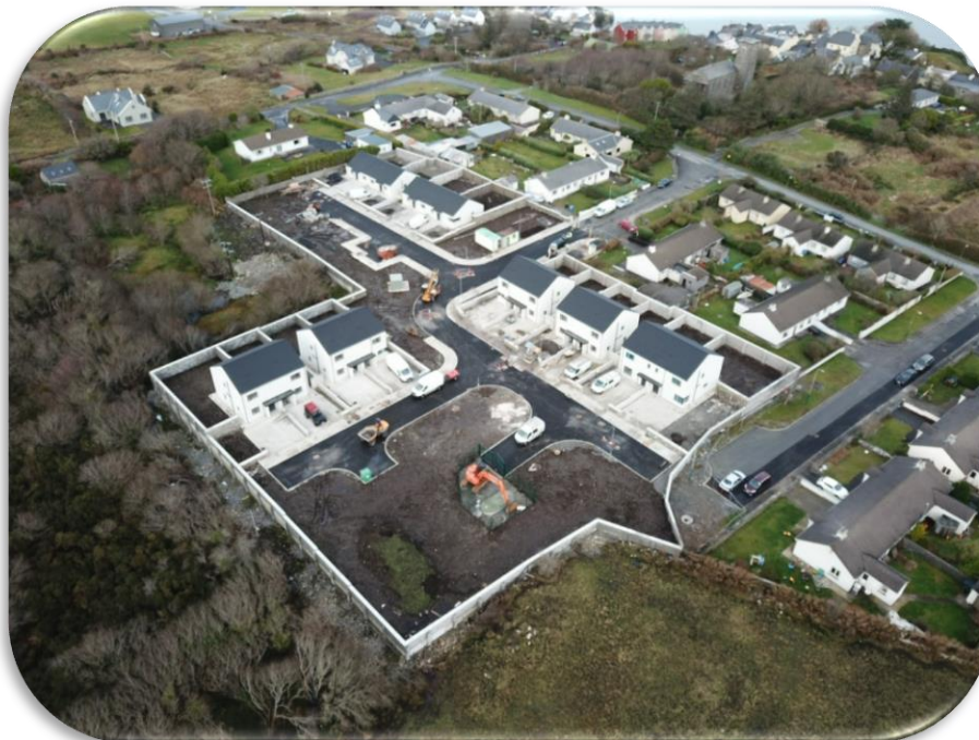
Cnoc na Carraige, Roundstone – under construction
