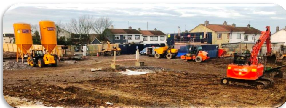
Fána Bhuí, Tuam – under construction
