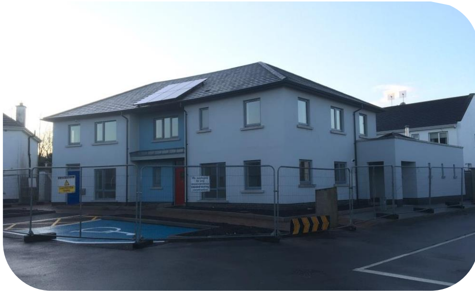
Finishing Disability Access Units – Esker Fields, Ballinasloe
