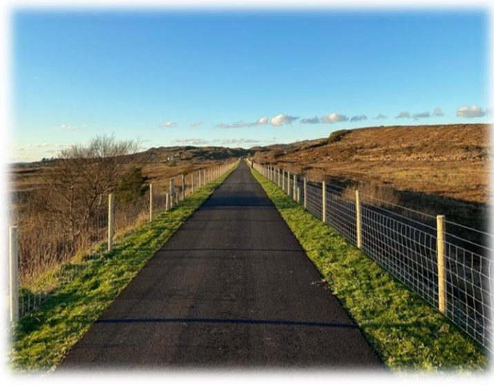
Connemara Greenway at Derryvickrune & Gowlan
