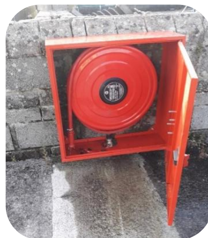
Fire Hose Reels Installed at Tuam Halting Site
