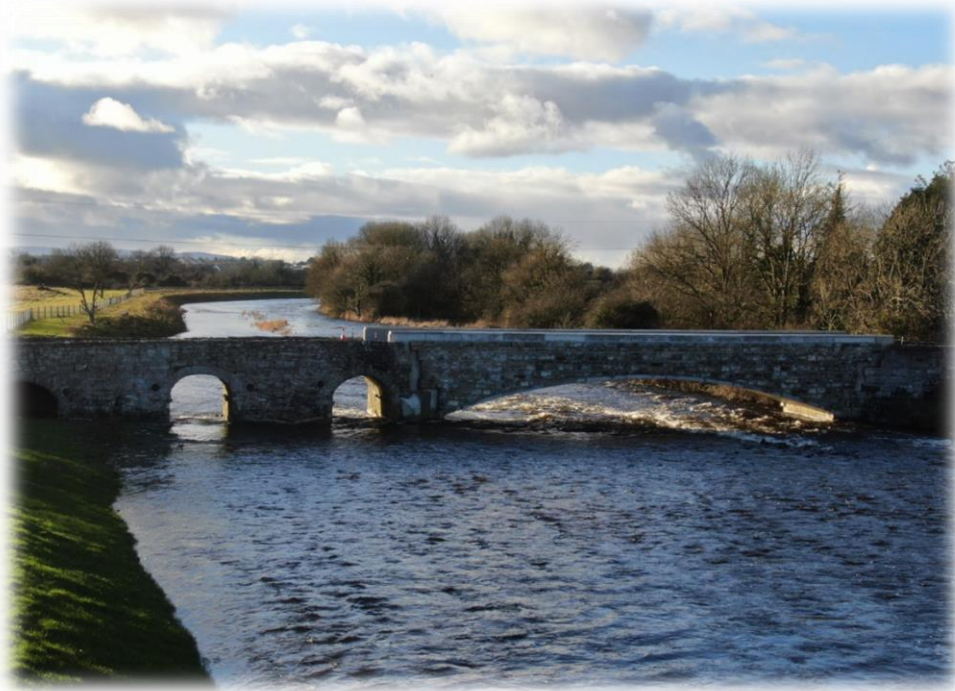
Dunkellin River & Aggard Stream Flood Relief Scheme – Completed Works at Dunkellin bridge
