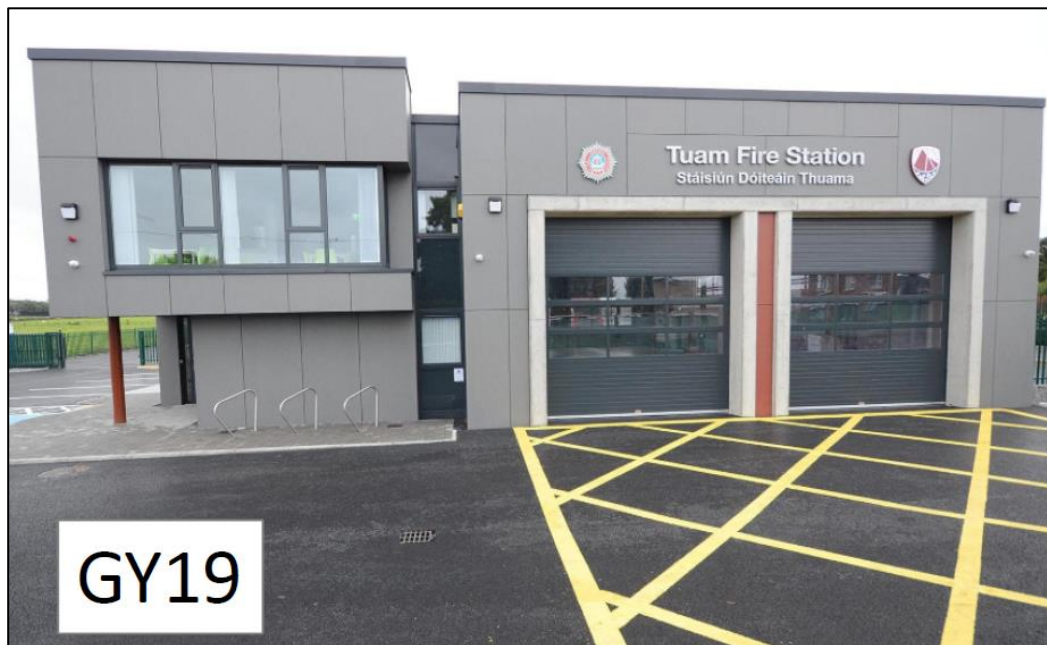
Figure 2: New Fire Station in Tuam Operational October 2018
