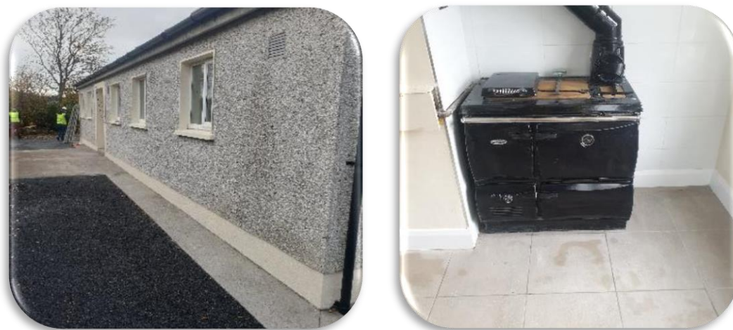
Major renovation works completed at traveller specific accommodation at Canal Drive, Ballinasloe
